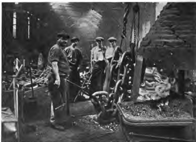
FIG. 354.—Welding link of Chain Cable for Super-“ Dreadnought.”
